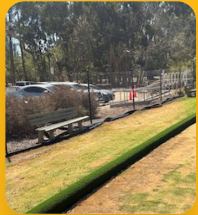
East facing cyclone fence by the entrance
